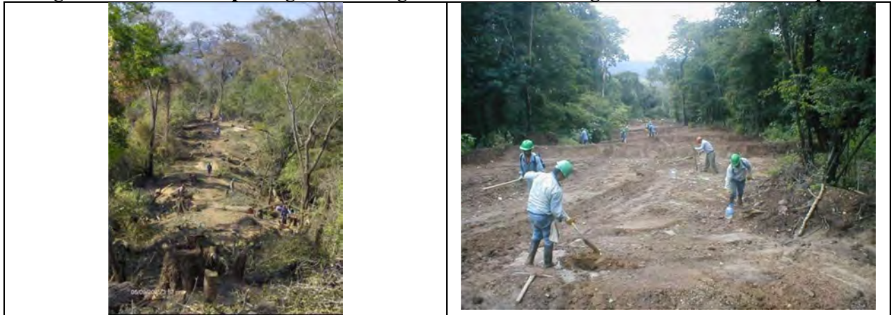
Figures 5a and 5b. Opening and closing narrow ROW using labor intensive technique 83
