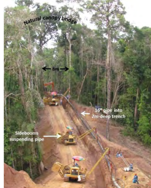
Figure 7. 8-meter construction RoW 86
