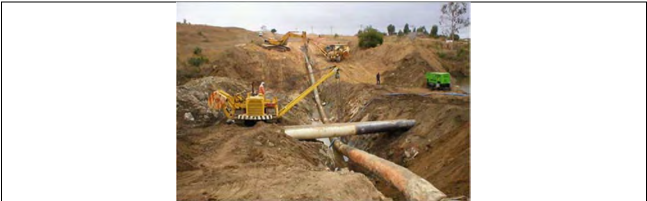
Figure 9. Open-cut pipeline crossing, horizontal pipes above pipeline for water flow 88
