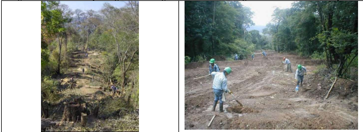
Figures 6a and 1b. Opening and closing narrow ROW using labor intensive technique 49
