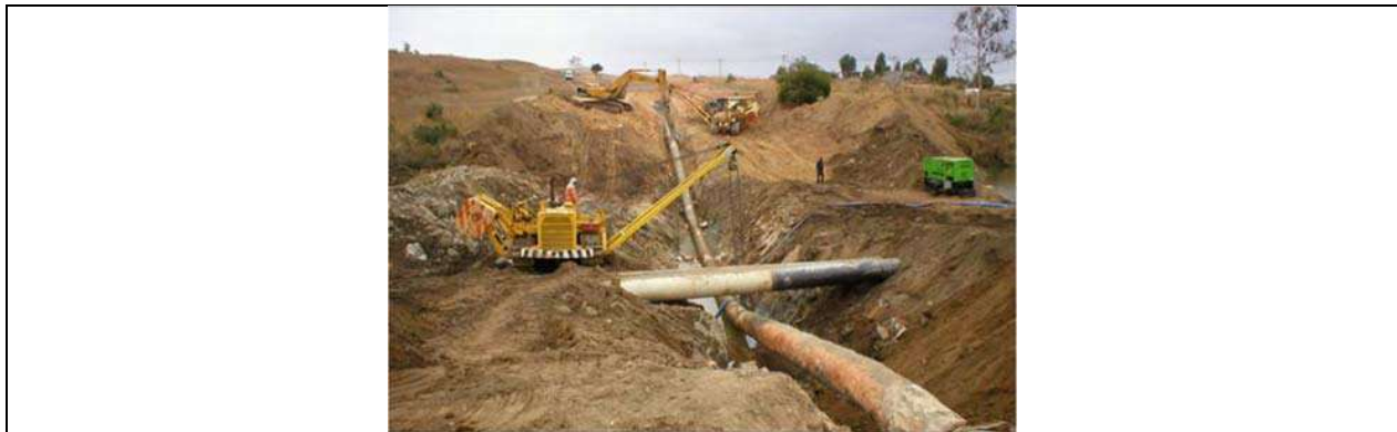
Figure 9. Open trench pipeline river crossing, horizontal flume pipes above pipeline for water flow 56
