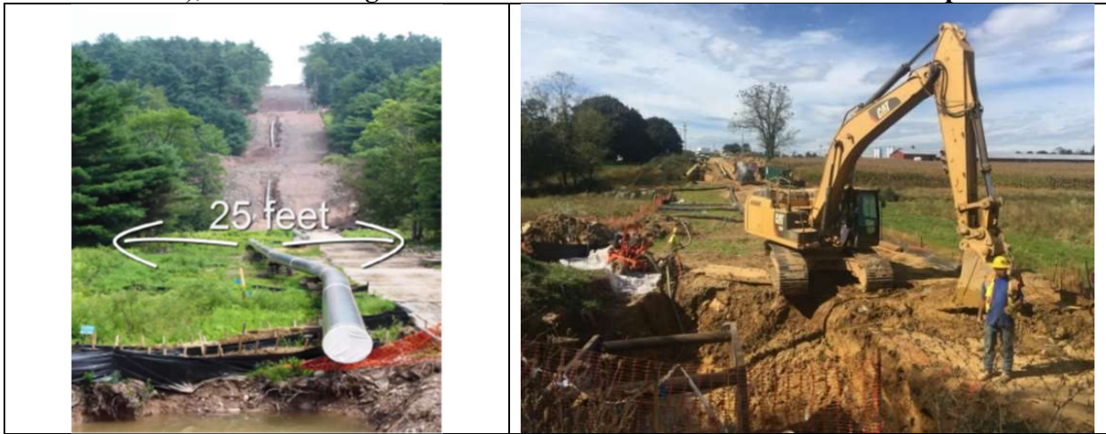
Figures 7a and 7b. Typical Pennsylvania 15-meter pipeline ROW (25 feet on either side of centerline), 50 and clearing of ROW for 20-inch diameter Mariner East Pipeline 51
