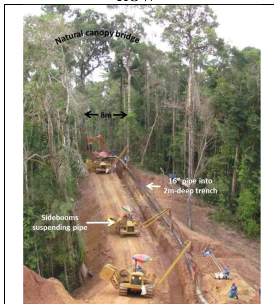
Figure 8. 8-meter construction ROW 53
